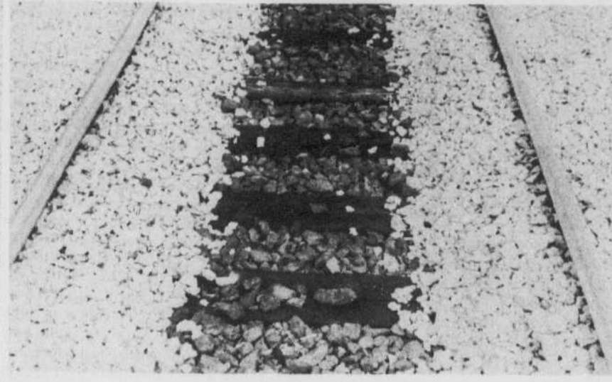
New ballast has recently been mixed with the older, asbestos-contaminated variety along a 2 km stretch of tracks near Abercorn.
