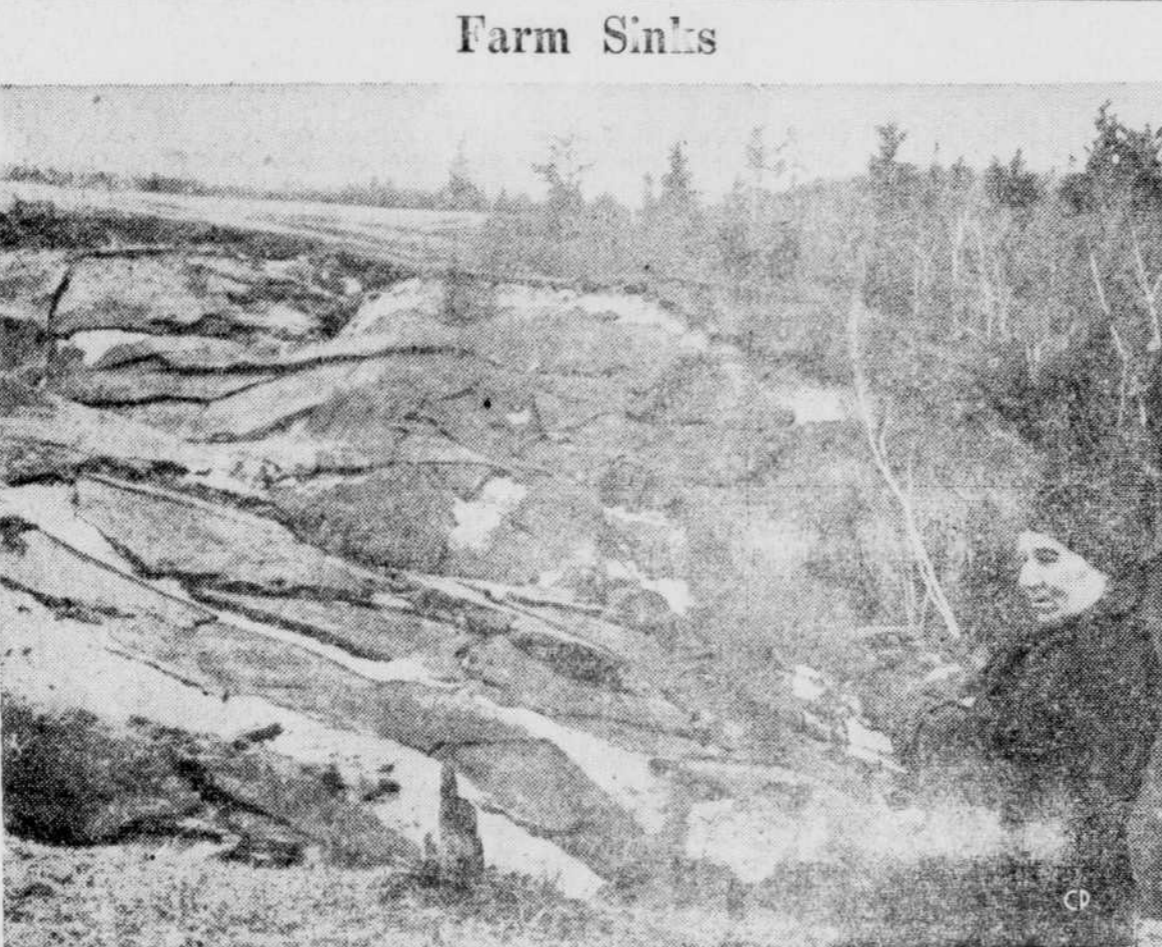
This caved-in section of a 20-acre farm is viewed sadly by Mrs. Leo Guglyk, wife of a Ukrainian farmer in the Espanola district of Northern Ontario about 50 miles west of Sudbury. During the last few weeks, almost all the land the elderly couple cleared from the bush 34 years ago has sunk, in some places as much as 65 feet. The sinking is believed caused by erosion from an underground stream. Advised to vacate their home, Mr. and Mrs. Guglyk say they have no place to go.
