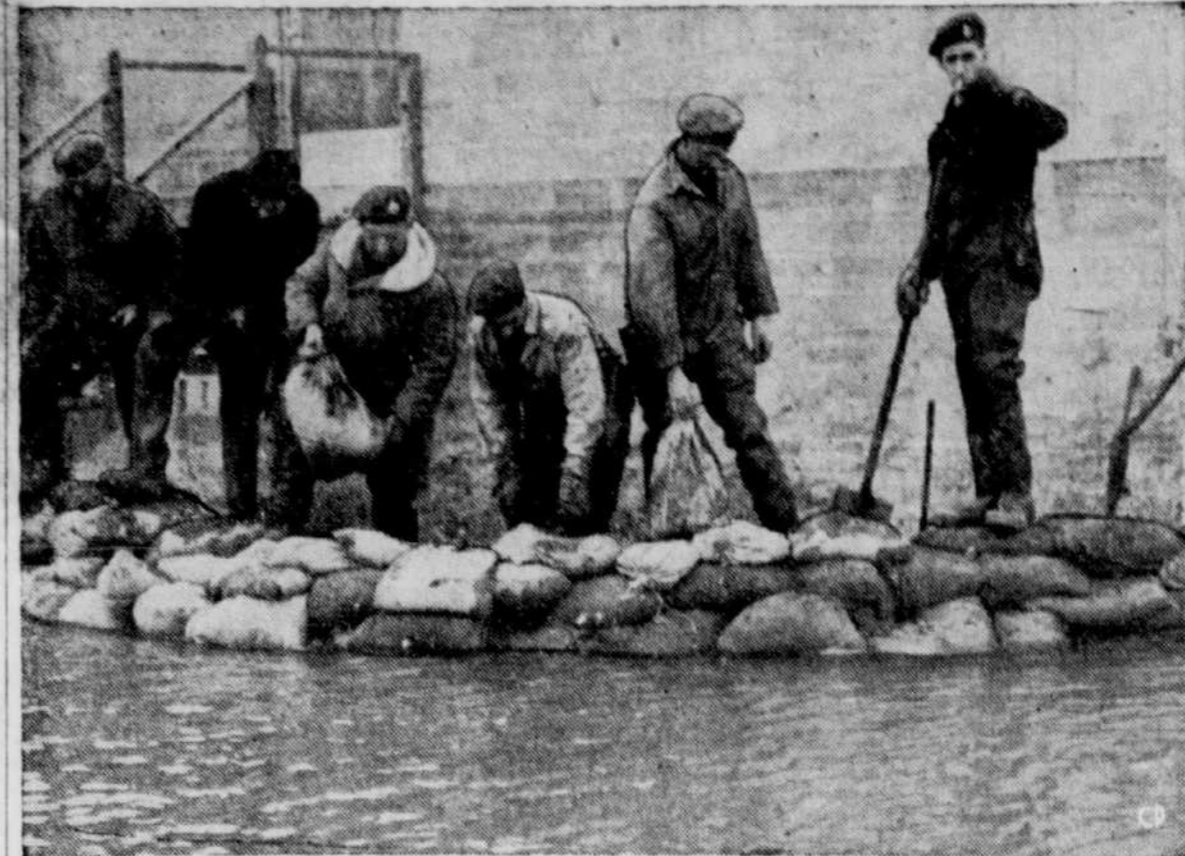
Soldiers of the Winnipeg area took over dyking operations when civilian workmen became exhausted, and kept flood waters from forcing seriously-ill patients and expectant mothers from the hospital at Morris, Man. By Monday morning, the soldiers had strengthened the dyke and increased its height above the level of the flooding waters. (P Photo)
