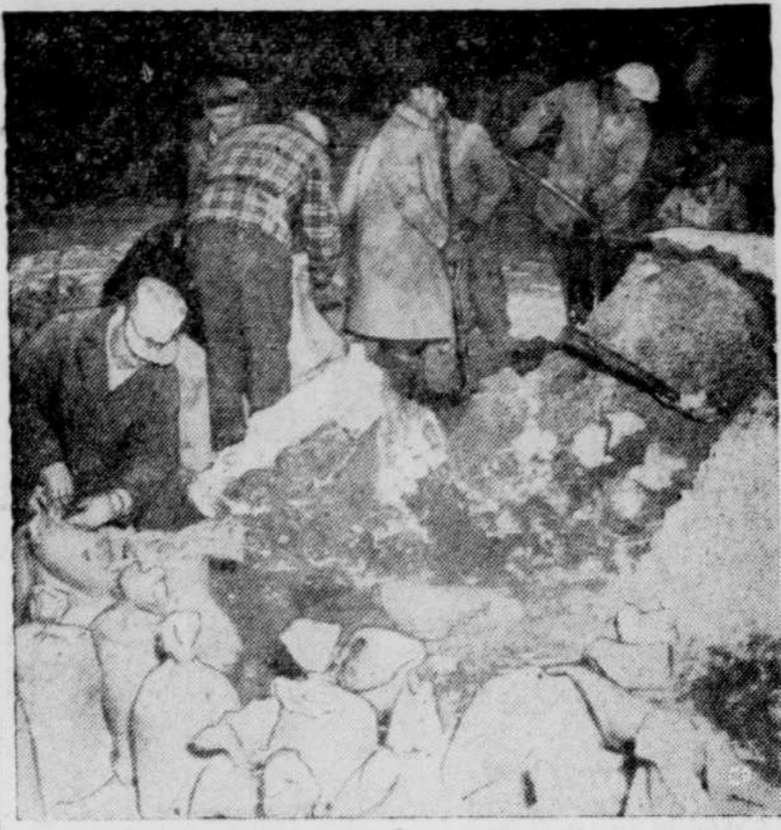
Volunteer crews in the Elm Park district of suburban Winnipeg were forced to fight wind-driven snow as well as flood waters from the Red River. Here they are erecting sandbag barricades in low-lying sections. They are a few of many fighting floods in the Winnipeg area.
