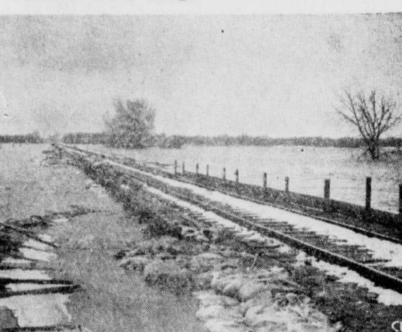
This Canadian Pacific Railway line across Bradley Coulee near Emerson, Man., faces the threat of being cut by floods. The swollen Red River was within six inches of the rail Thursday. Normally water is 20 feet below the top of the rails. Railway officials think the track, running across a long fill and reinforced with 60 cars of gravel, will not wash out.
