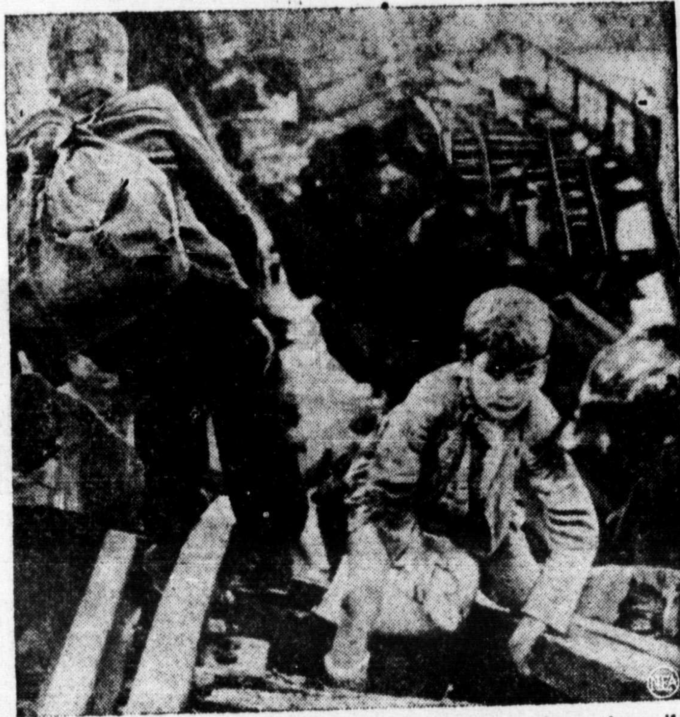
Two French boys are shown climbing over the wreckage of a railway bridge on the Moselle river to recover food supplies from railroad cars which were on the span when it was destroyed by Germans retreating before Allied forces.
