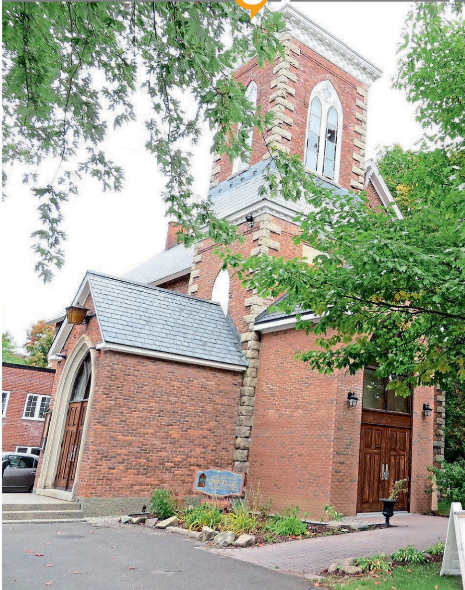
Emmanuel United Church is located at 203 Principale in Cowansville. (Photo: courtesy)
