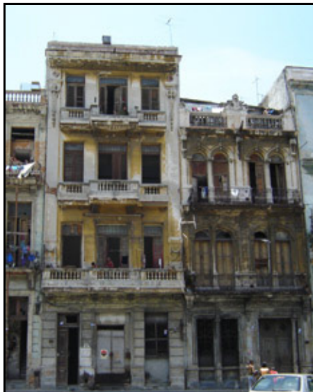
Figure 1.59: Buildings falling apart.
