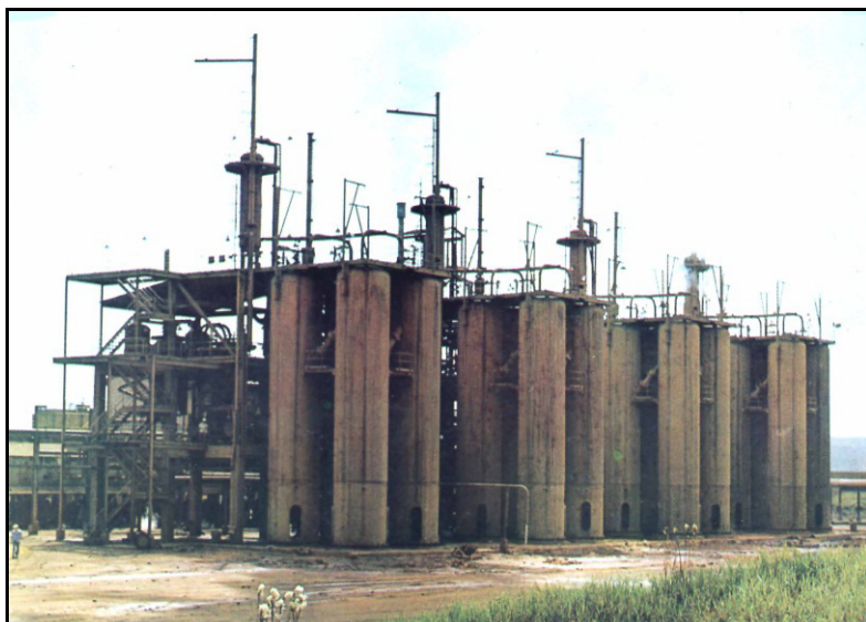
Figure 1.41: Leaching autoclaves for laterites in Moa.
