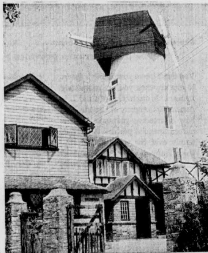
OLD MILL AND COTTAGE , Battle, Sussex — Old mills are still to be seen in Britain, but although many of them are kept in a good state of repair like this one, few retain their sails and have retired from their original task of grinding corn. (British Travel Assn.)
