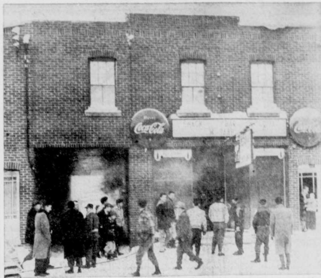
RICHMOND BLAZE — Fire breaking out in the cellar of the Rahal Restaurant, Main street, Richmond, caused smoke damage to the store and the upstairs apartments occupied by Mrs. Mabel Blanchette and Mr. and Mrs. Reginald Patrick. Firemen under Chief Gerard Paquin and Assistant Chief Leslie Rattray quickly controlled the outbreak. (Record Photo by Wm. H. Lunan)
