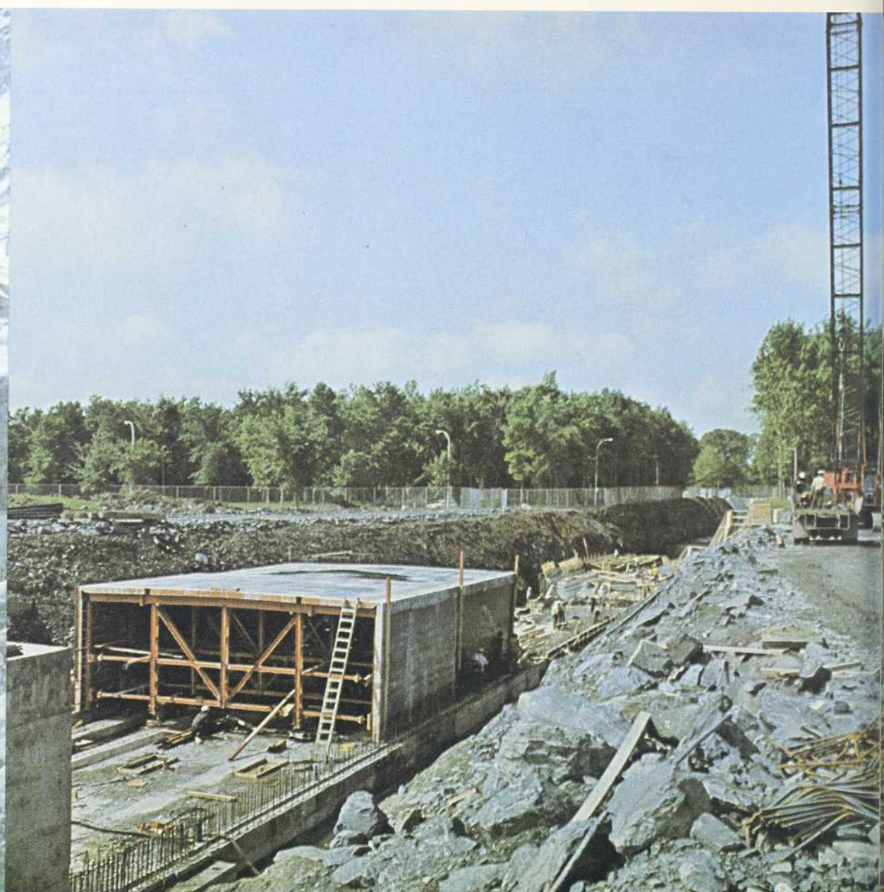
ANGRIGNON REAR STATION AREA
