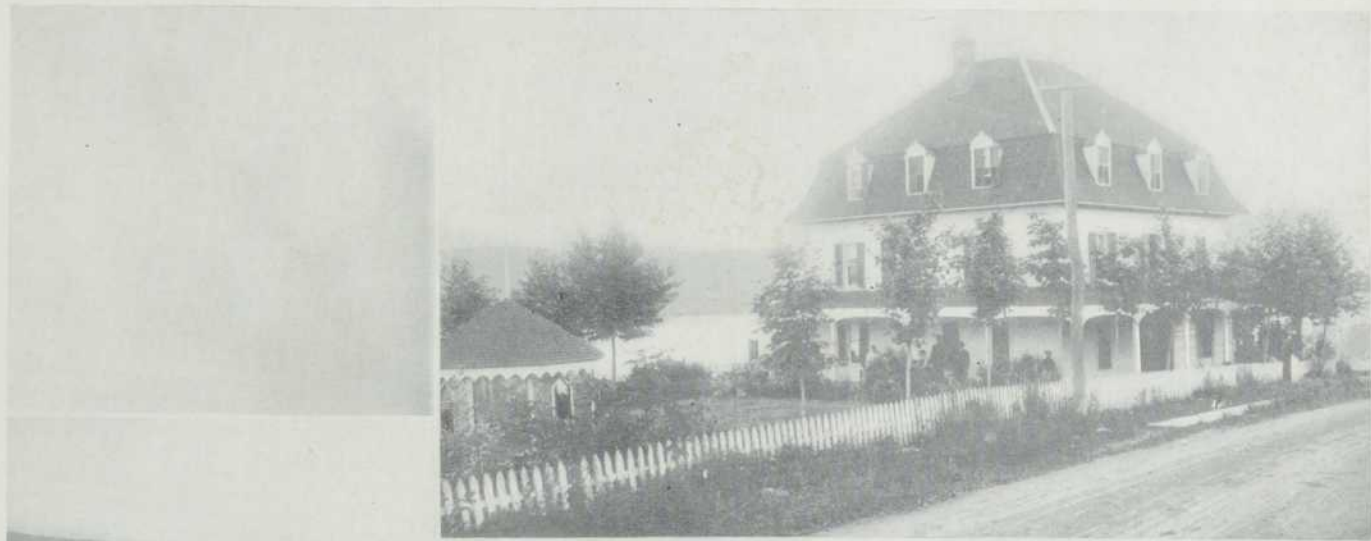
Cloutier Hotel, on the Line of the Temiscouata Railway.
