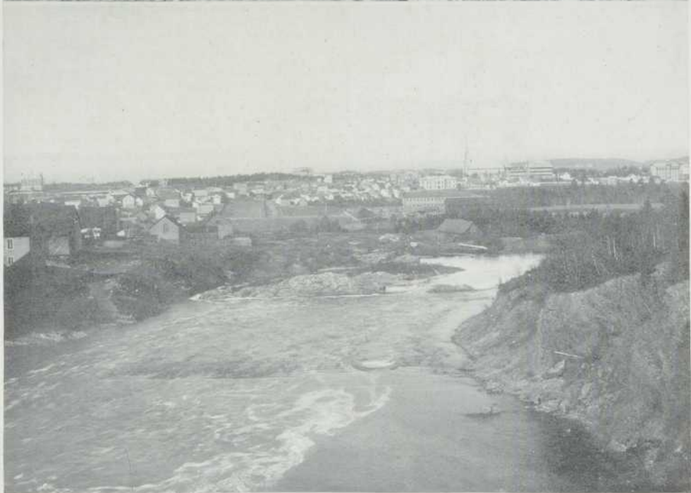
View from I. C. R. Bridge.
