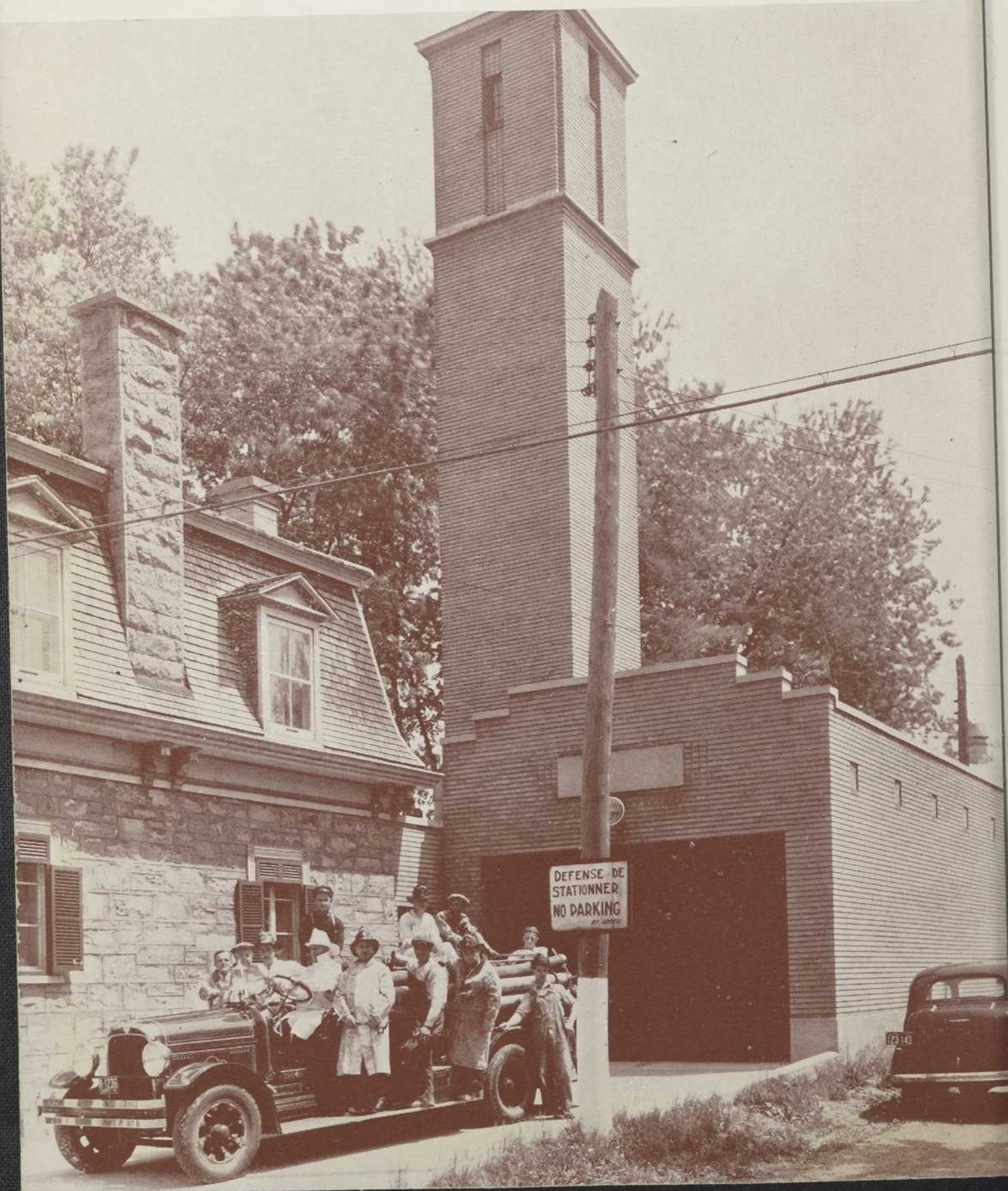
Station de pompes de Sainte-Rose
