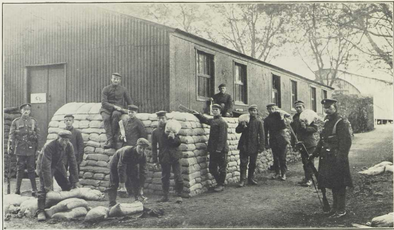
GERMAN PRISONERS OF WAR SANDBAGGING ONE OF THE HOSPITAL HUTS TO PROTECT THE OCCUPANTS DURING ENEMY AIR RAIDS
