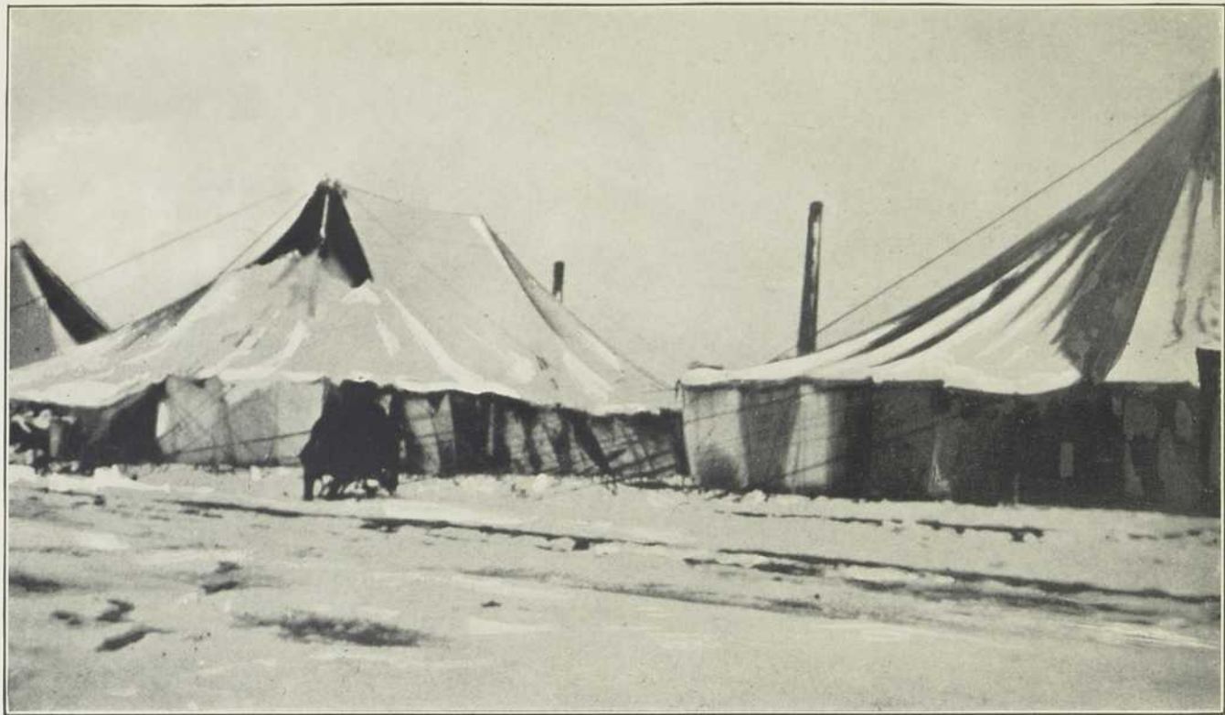
DAMAGED TENTS OF NO. 3 HOSPITAL, DANNES-CAMIERS, AFTER THE GREAT SNOWSTORM OF NOVEMBER 13, 1915
