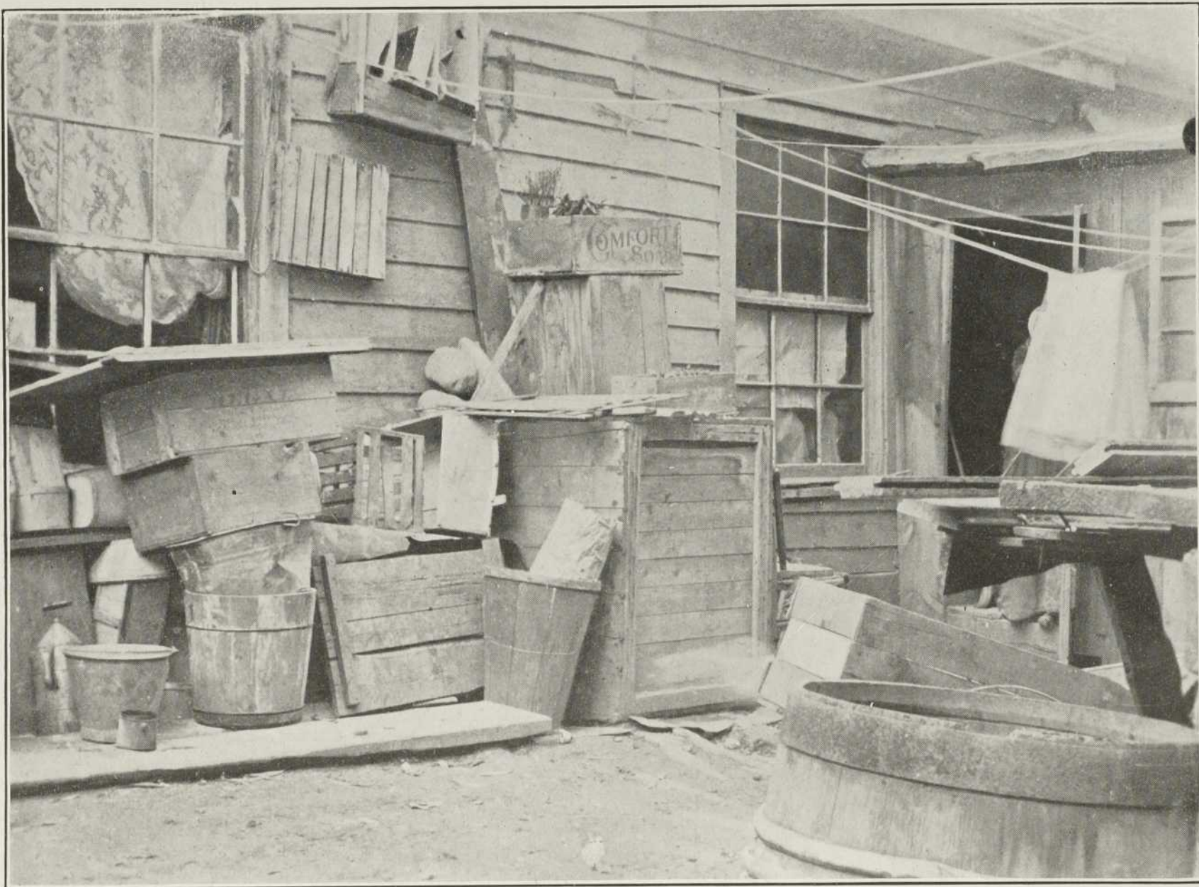
Too much rubbish in evidence.
