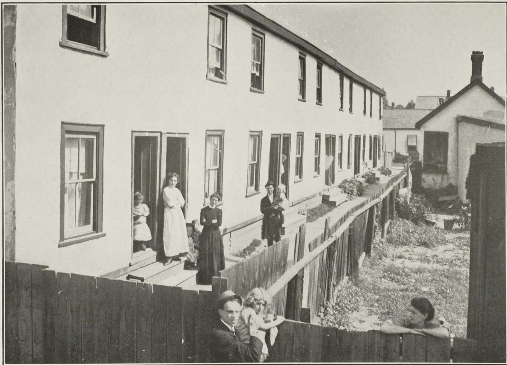
Houses built in lanes and alleys all too common.
