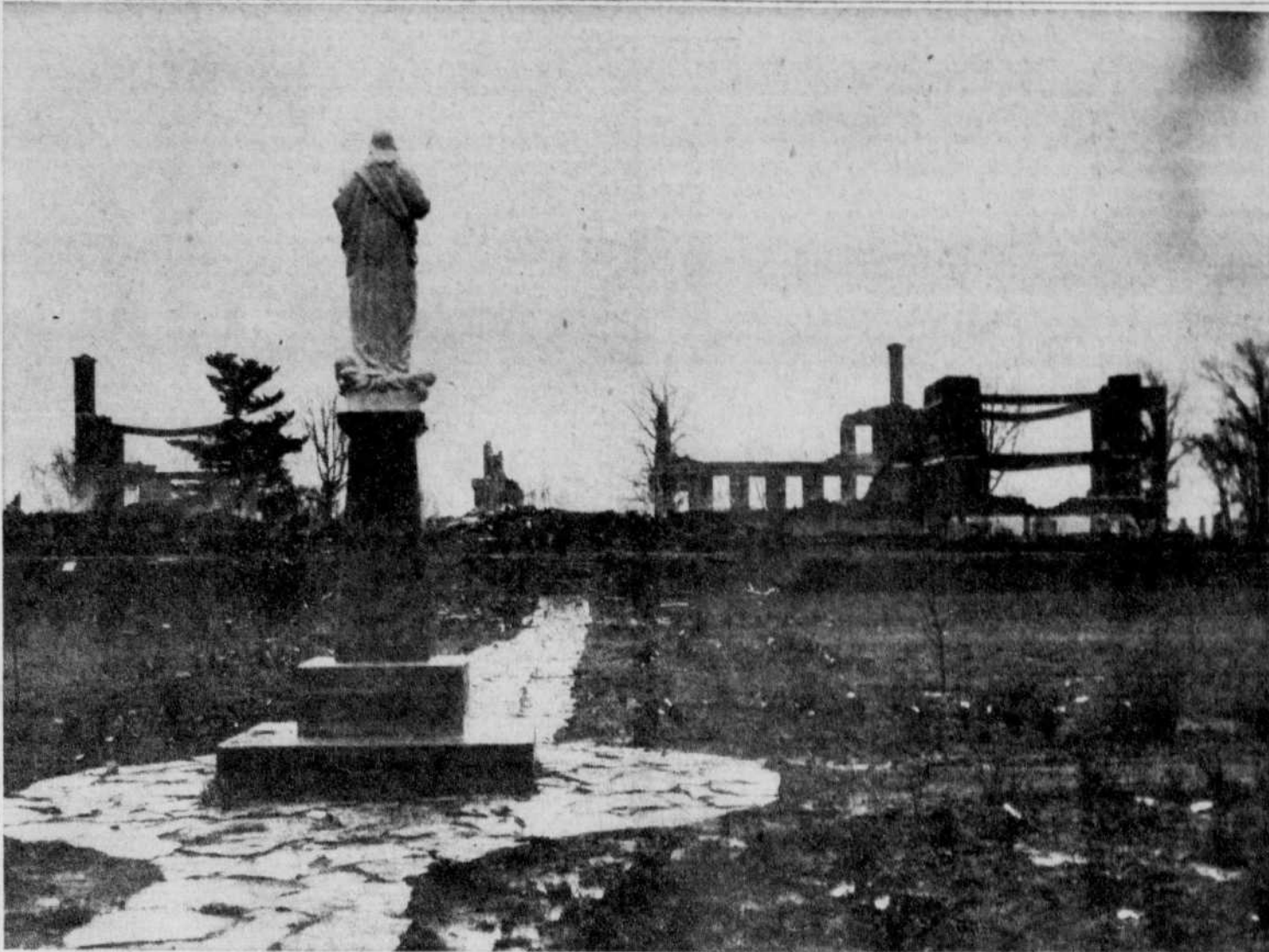
Symbol Of Faith — The statue of the Grey Nuns is the only standing object in the convent grounds near Ottawa. The blast that levelled the building behind was caused by a crashing CF-100 jet fighter of the RCAF. Fifteen died.
