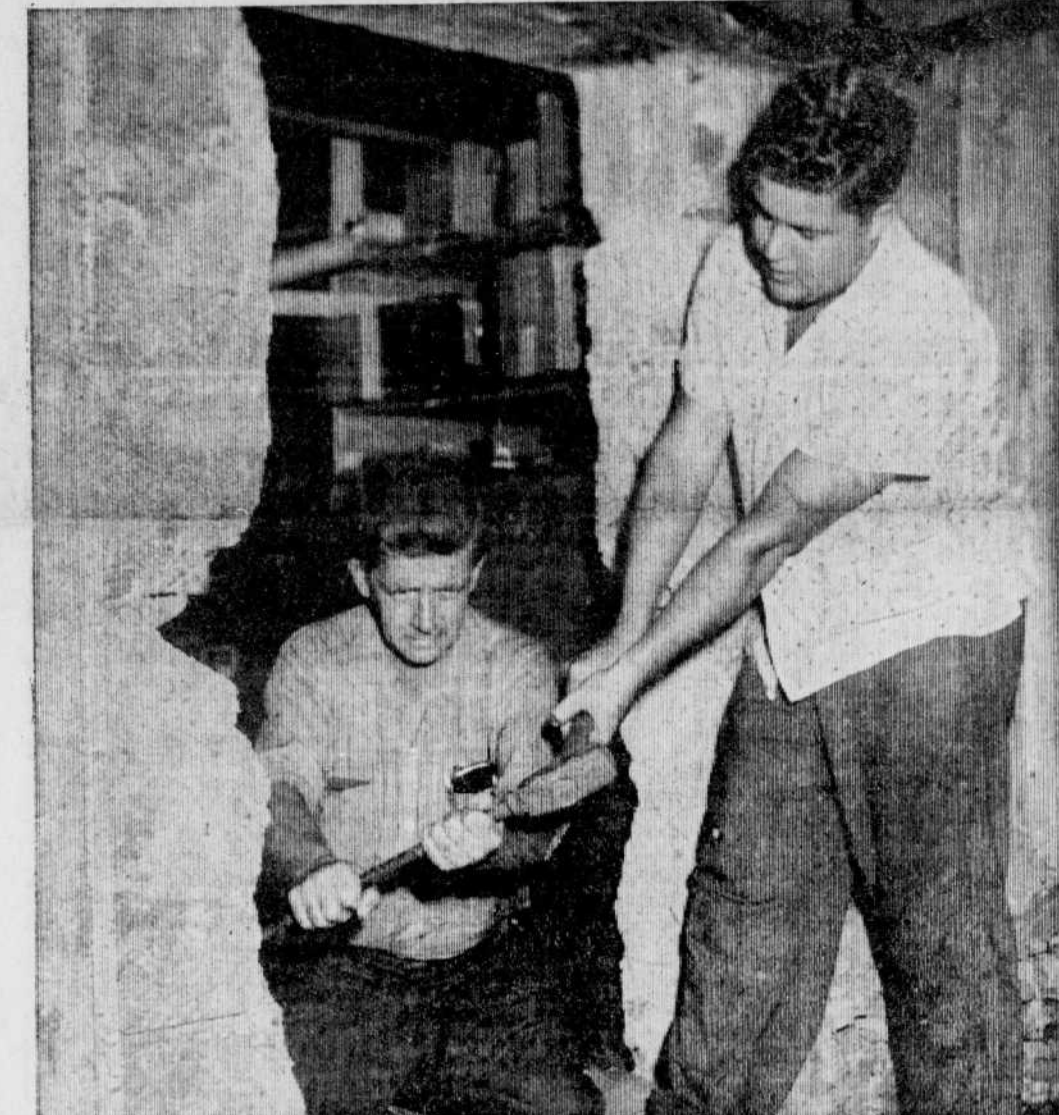
FALLOUT SHELTER UNDERWAY — Work is moving swiftly on construction of a fallout shelter at the home of Armond McBurney in Sawyerville. Upper photo shows Mr. McBurney digging out one-end of the concrete-enclosed structure. The roof above his head is composed of nine inches of steel-reinforced concrete. In the lower photo, Mr. McBurney (left) and his son James square off the entrance to the shelter, which is being built adjacent to the basement of his home. The shelter should be ready for an emergency by this fall. (Record photos by Gerry Lemay)
