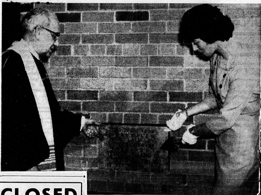
AT CORNERSTONE LAYING: RABBI DR. HARRY J. STERN of Temple Emmanu-El, and Mrs. Sytaey Lithwick, representing Hyman Grover, president of the congregation, officiate at the cornerstone laying of the new addition to the Temple.
