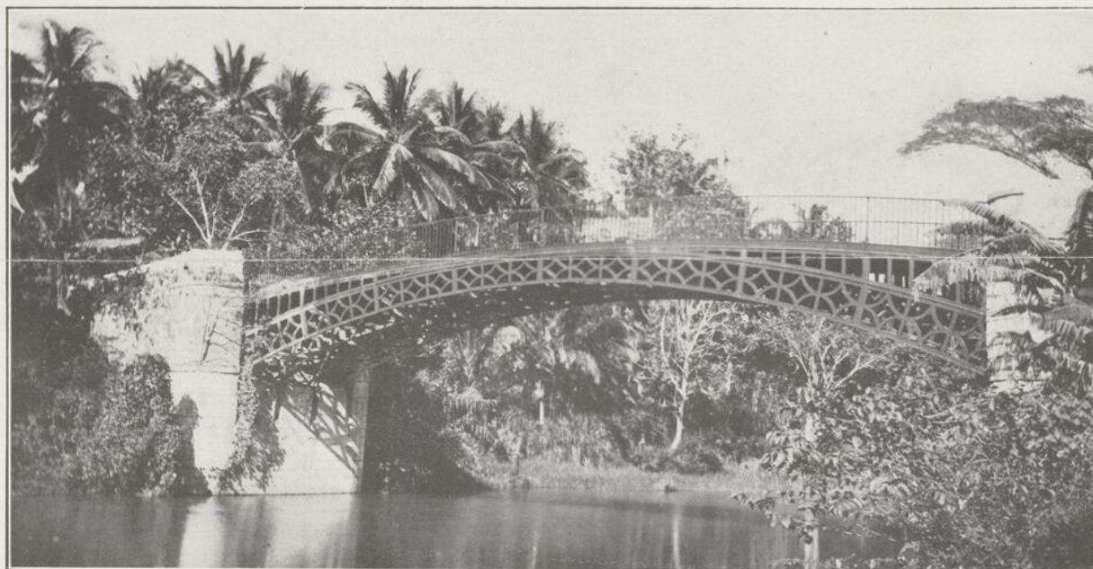
BRIDGE OVER THE RIO COBRE RIVER, JAMAICA—This structure is noted for the beauty and grace of its design. It stands in the midst of beautiful scenery.
