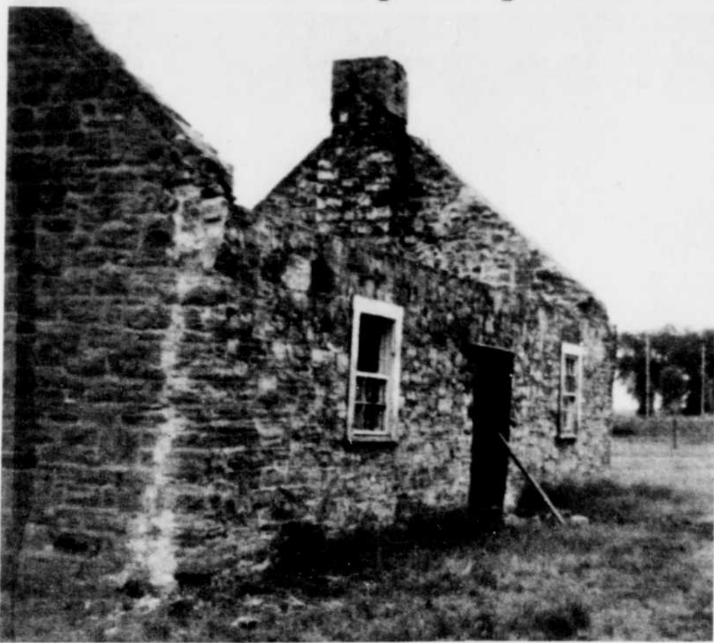
SOON COMPLETED — The restoration of this building on the Macdonald College farm will soon be completed and two Eastern Townships youths are playing a large part in
