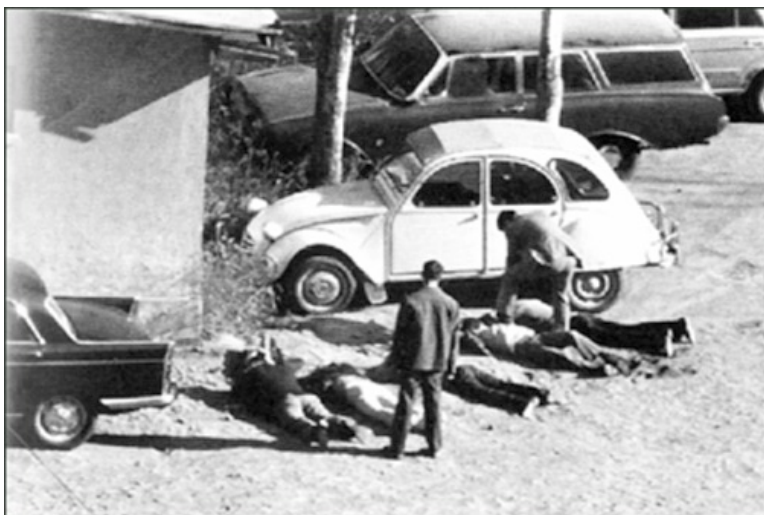
Photo by Christian Montecino Chile From Within People arrested after trying to enter the embassy of Argentina 1973
