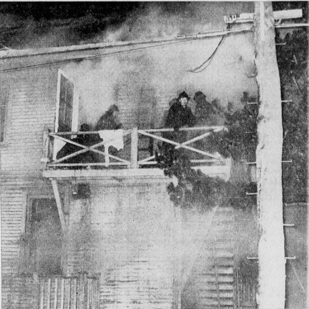
MAGOG FIREMEN COMBAT BLAZE — Firemen from the Magog Fire Department are pictured on the balcony of this four-story tenement house which was badly damaged by fire late Saturday afternoon in Magog. The blaze started as a chimney fire and simmered for several hours before finally spreading through the whole house. (Record Photo by Charles Catchpaugh)
