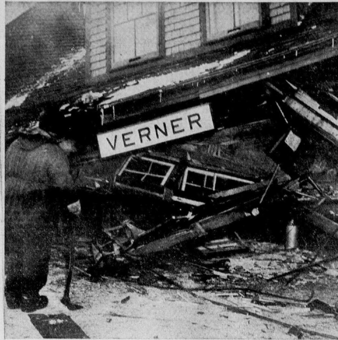
NO TRAINS TODAY — The frame CPR railway station at Verner, Ont., a village of a few hundred, 44 miles east of Sudbury, had one end reduced to little more than a pile of lumber Friday when a west-bound freight hit an open switch, sped down a dead-end spur and catapulted two empty boxcars into the building. The boxcars had been shunted to the end of the spur when the train, loaded with newsprint hit them. Station Master Rejean Lafreniere, of Ville Marie, Que., was inside the building when the train hit the switch and realizing the impending danger ran outside seconds before the boxcars smashed into the building. There was one slight injury. (CP Photo)
