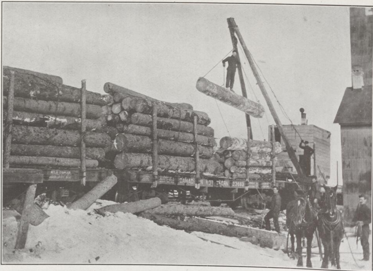
LUMBERING IN MANITOBA—Loading logs at Minitonas for shipment to Mafeking.
