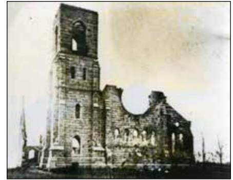
1. Centenary United Church after the fire in 1883 (ETRC, UC011 Centenary United Church fonds)
