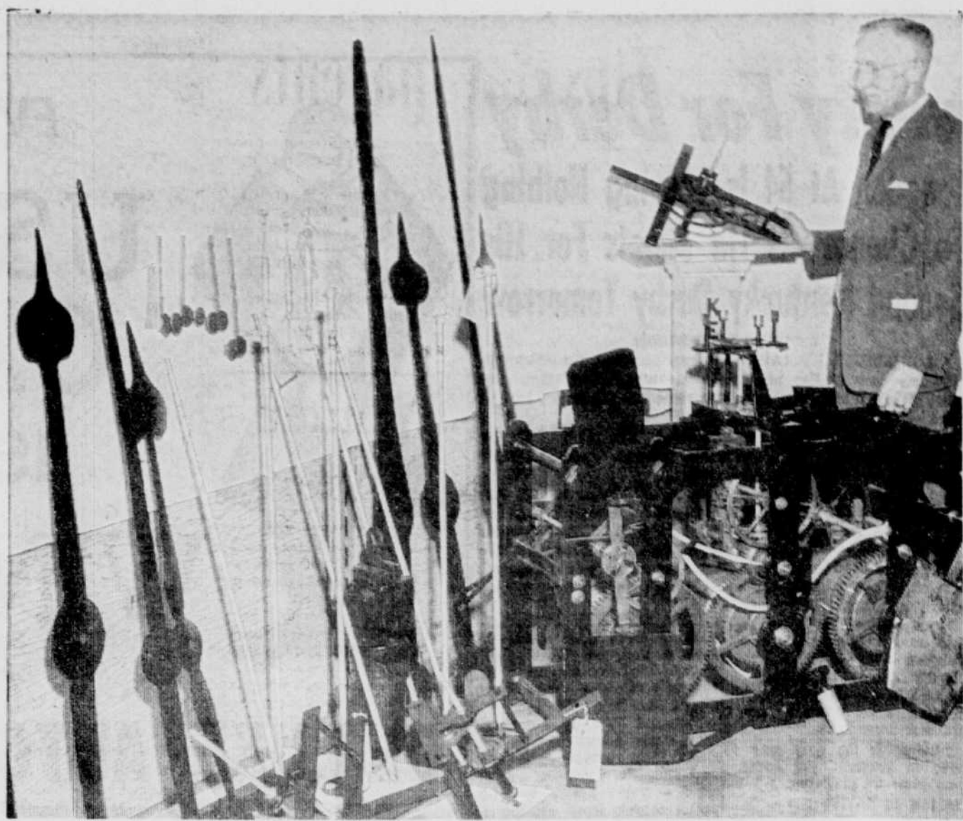
HALIFAX TOWN CLOCK — It looks confused but watchmaker Clem Hughes will soon have the Halifax's historic old town clock in running order. The 166-year-old clock was taken apart last year for its first repair job in more than 1½ centuries. Those wicked-looking spears against the wall are the eight hands of the four-sided clock. (CP Photo)
