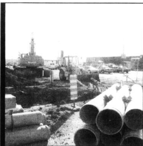
Construction work is progressing at the Galeries d'Ormstown site. (Photo: JT)
