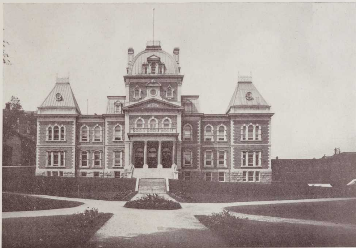
COURT HOUSE AND STRATHCONA SQUARE
