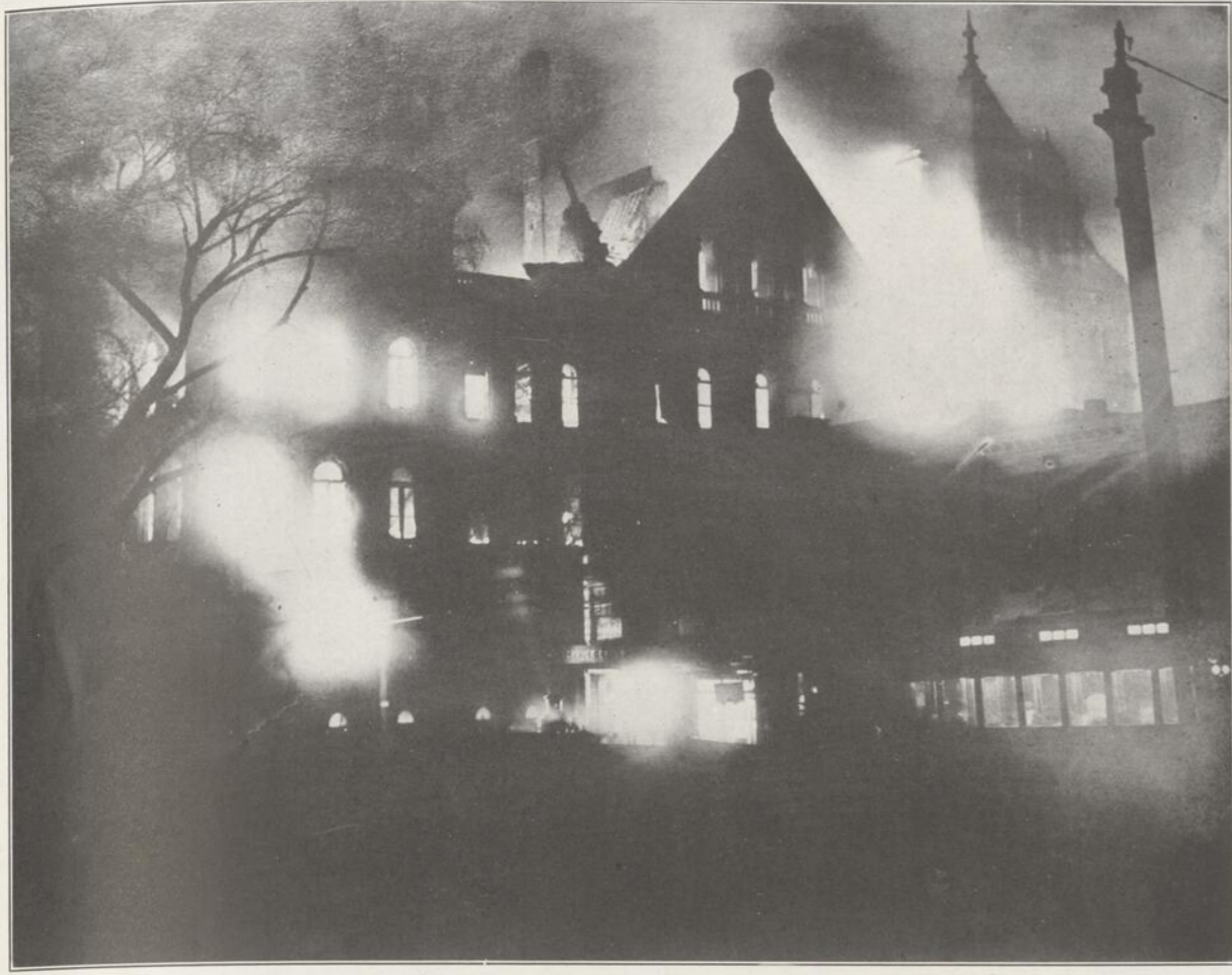
THE RECENT FIRE IN THE STATE CAPITOL AT ALBANY, N.Y.—A view of the conflagration from a photograph taken at 3.30 in the morning. This photograph was made from the new educational building on Washington avenue, and shows the whole rear of the capitol, and the chimney that ran up through the roof above the State Library in the centre of the building. The high tower seen to the right fell about 5 a.m. The high tower dimly seen in the north-east was burning fiercely at 10 a.m., and fell shortly after. The State Library is between this tower and the high tower to the right. (Photo by Underwood and Underwood.)
