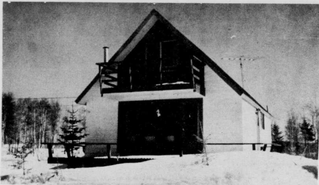
WINTERIZED FOR YEAR 'ROUND — The Halliday chalet shown here was first designed as a year 'round second home, but like many cottages, was winterized and finished as a permanent home.
