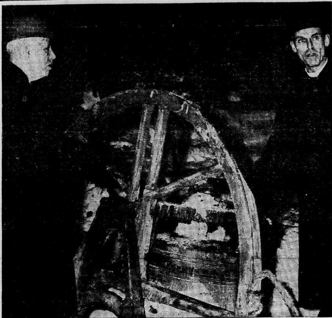
The City of Valleyfield has started the demolition of the remains of St. Mark's Anglican Church in Valleyfield this week and one of the first things that had to be done was to remove the bell from the belfry in the church tower. As its contribution to rebuilding the church the city is doing this work free of charge. Here we see Rev. John Hall, right, and Mr. C. Gurnham with the bell in front of the church after it had been taken down by a large crane. The bell was cast in 1850 and was first used in St. Georges church in Montreal before being moved to Valleyfield. (Photo - Peter Rozon)
