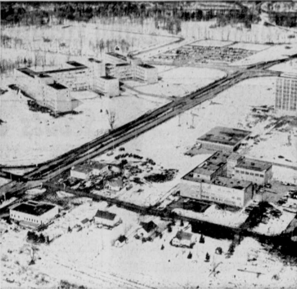
MOVE FEDERAL OFFICES — The federal government is moving out of some of its cramped office space in downtown Ottawa to Confederation Heights, four miles south of Parliament Hill. This aerial view of Confederation Heights shows the Sir Charles Tupper public works and fisheries department headquarters (left), public works testing laboratory (right foreground), post office headquarters (right centre) and National Research Council communications headquarters (right background).
