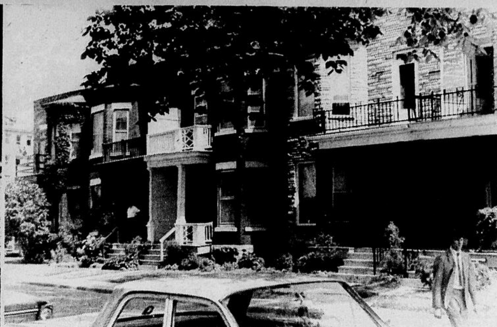
Typical homes on nearby Burton avenue.
