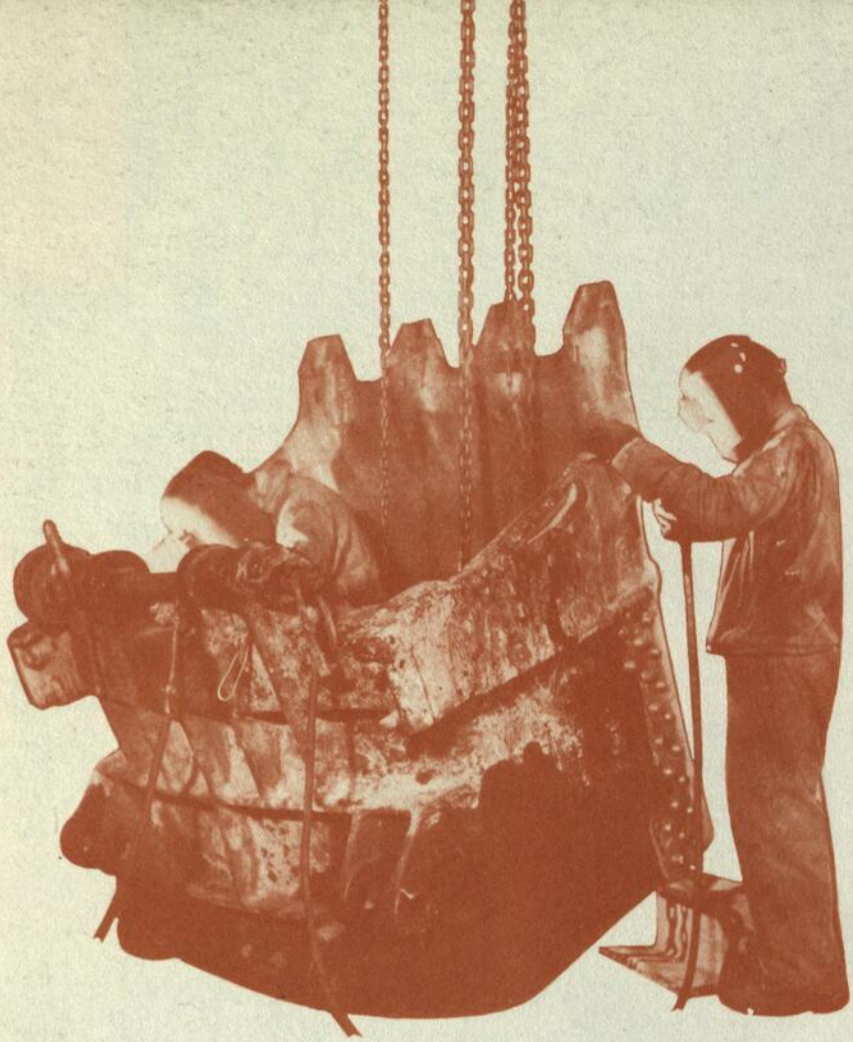
Welding teeth on a shovel bucket. Facilities for major repair jobs were maintained at Sept Iles and up the line at Miles 224 and 290. Heavy equipment airlifted north was frequently cut apart for shipment and welded back together in the field.
