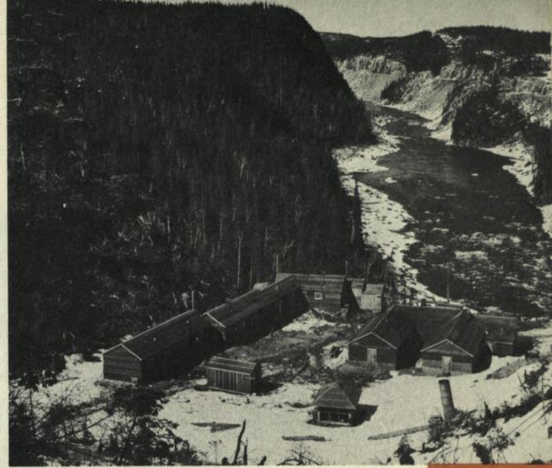
The Moisie River brawls its way through this canyon above the camp at Mile 12. Railroad bed cut into solid rock can be seen clinging to cliff wall at right.
