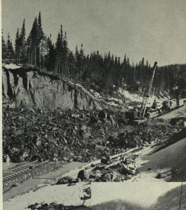
Mud and rock plagued builders constantly. (above) Crane works to clear a slide of silty clay, 75 yards long, 20 feet deep, off track at Mile 11. (right) Wreck crew clears derailment caused by rock slide.
