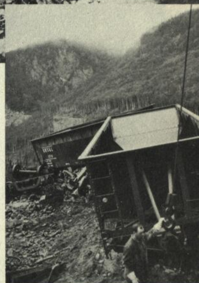
Mud and rock plagued builders constantly. (above) Crane works to clear a slide of silty clay, 75 yards long, 20 feet deep, off track at Mile 11. (right) Wreck crew clears derailment caused by rock slide.
