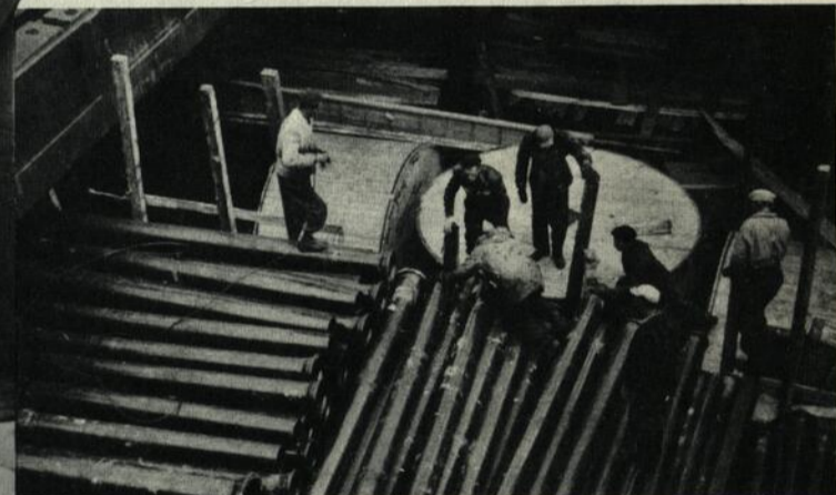
Unloading pipe at Sept Iles. Iron Ore Company purchased its own 2500-ton vessel, the S.S. Easton, to facilitate freight movement from Montreal.
