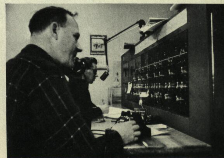
Dispatcher at Centralized Traffic Control panel directs trains, operates power switches and signals.
