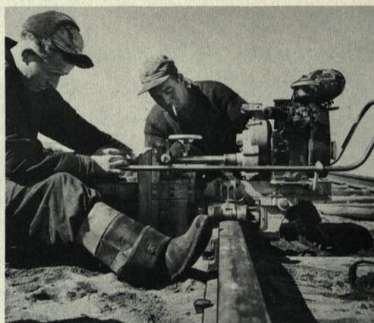
Gasoline-powered drill bores hole for bolt installation at joint.
