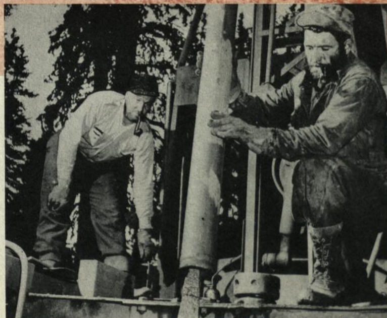
Removing a sample from a drill hole. Careful mapping made it possible to concentrate on likely areas; more than 2,700 tons of ore were indicated with each foot of drilling.
