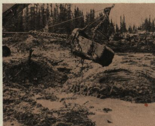
Muskeg along the line. In many places roadbed was built right over it. This muskeg will compress to 3 inches for every foot of depth. (left) Drainage ditch opened by propagation blasting. (right) Drag-lining muskeg.
