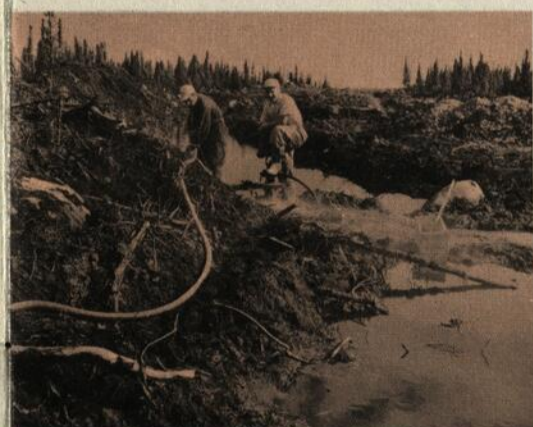
Muskeg along the line. In many places roadbed was built right over it. This muskeg will compress to 3 inches for every foot of depth. (left) Drainage ditch opened by propagation blasting. (right) Drag-lining muskeg.
