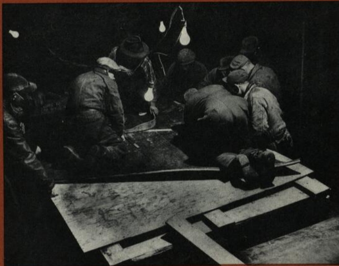
Splicing 60-inch belt under dumper at Sept Iles.
