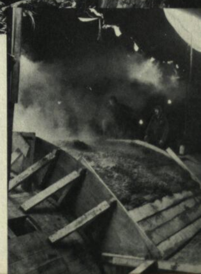
Break through near south portal of the 2206-foot tunnel at Mile 12; 100 thousand cubic yards of material flowed through this hole. Damage was repaired (right) by capping with concrete.
