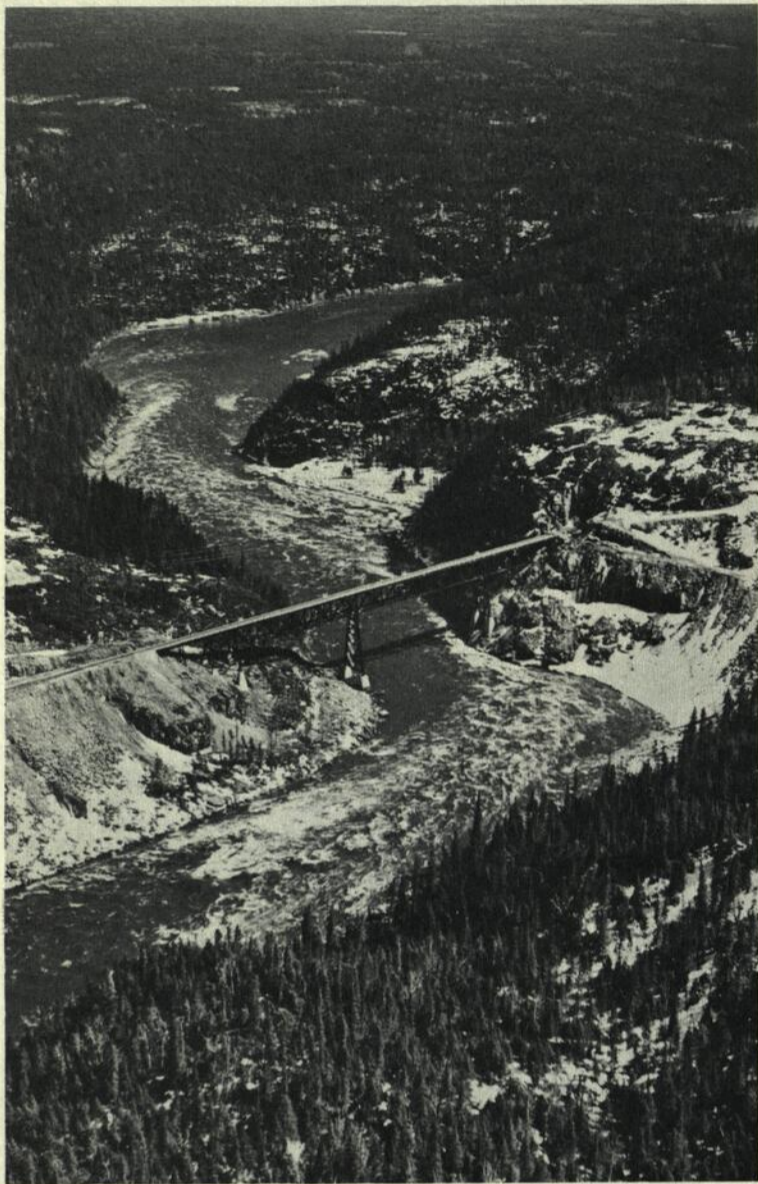
Longest bridge on the QNS & L, the 705-foot span at Mile 12 over the Moisie River has its south end at the mouth of a half-mile tunnel and its north end on a shelf of solid rock which had to be blasted to make room for the roadbed.
