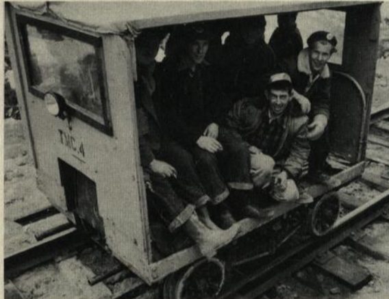
Speeders carry section hands from point-to-point along railroad as they put finishing touches on the track.
