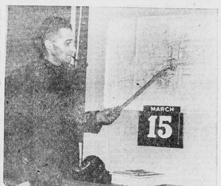
LEIGH BLADEN is engineer in charge of the work being carried out by Relocations Limited at Thetford Mines. (Record Photo by Gerry Lemay)
