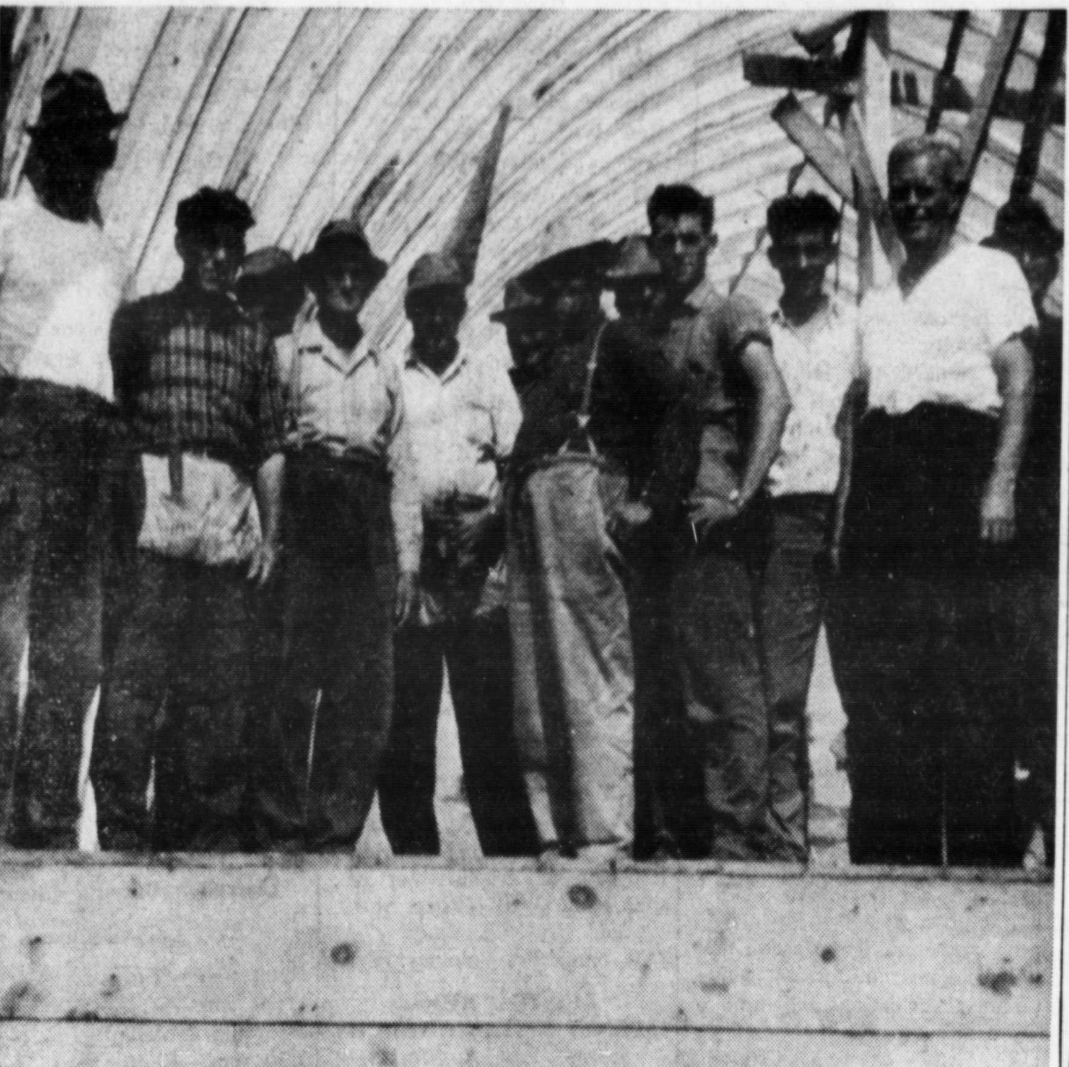
These are the men who built the Hall, being rafter, John Pepin, John Kavanagh, Pat Kavanagh, Father T. G. May, P.P. and Adolph Pepin. Others were up on the scaffolding when the above photo was taken.
