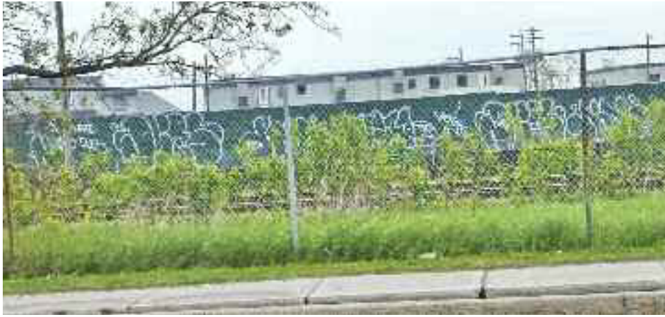
Graffiti-ridden plywood fence on Glen Yards hospital site, May 19
