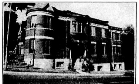
Westmount: Renovated, unique! $419,000 Barbara Bourke 871-8710
