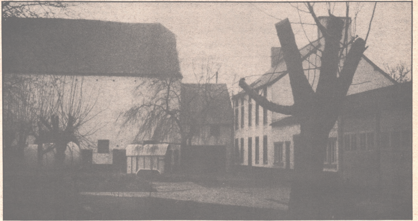
Mr. Barré's farm buildings are surrounded by a high stone wall. The stone house and barn encircle a courtyard and is paved in brick and cobblestone.
