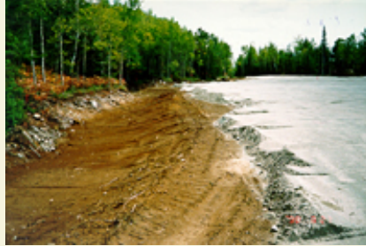
A multi-layer covering installed to control acidic mine drainage.
