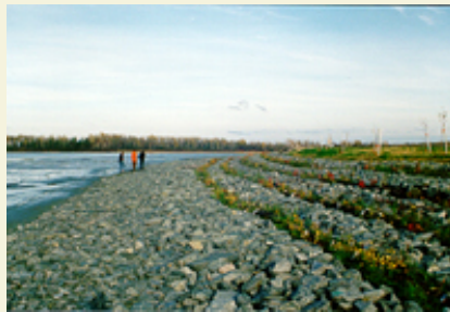
The bank stabilization join the mechanical and vegetal stabilization technics.
