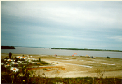
The same site, during the restoration work in 2000.
