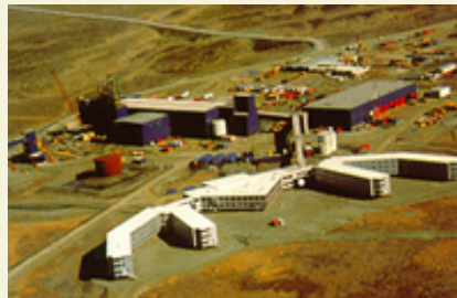
Raglan Mining facilities.
