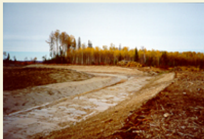
Excavation work for the "new" Ruisseau Pandora.
