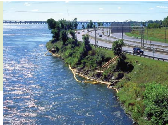
Figure 6.25 The Technoparc waterfront: highway facilities.
