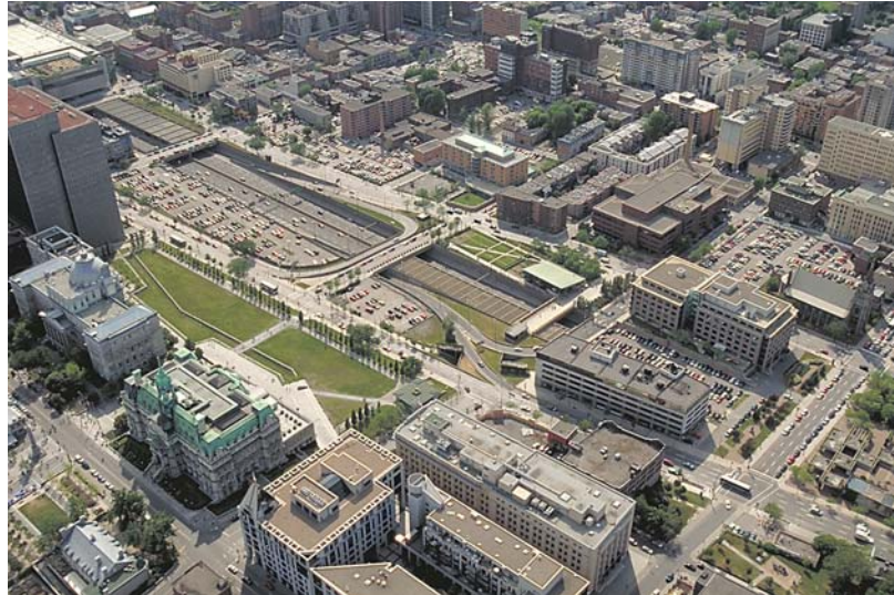
Figure 6.42 Ville-Marie Expressway trench north of Champ-de-Mars — development potential of more than 185,800 m 2 .
