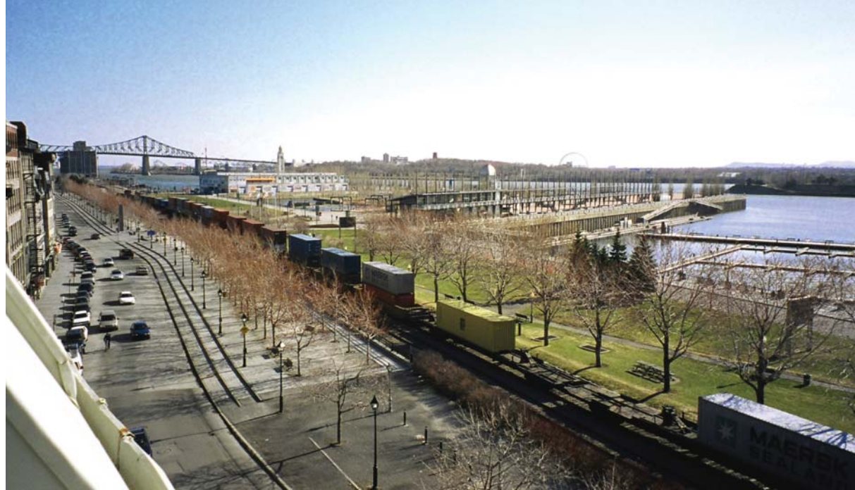
Figure 6.11 Old Port rail lines: uneasy cohabitation between old and new.
