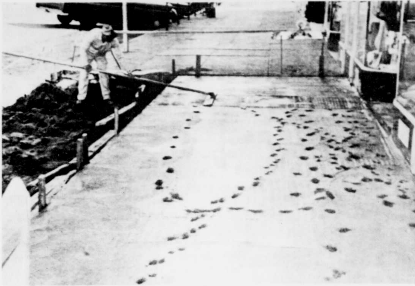
PAWS THAT REFRESHEN — Workmen had just finished pouring the concrete sidewalk in front of a downtown Enid, Okla., store and looked back to admire their work just in time
