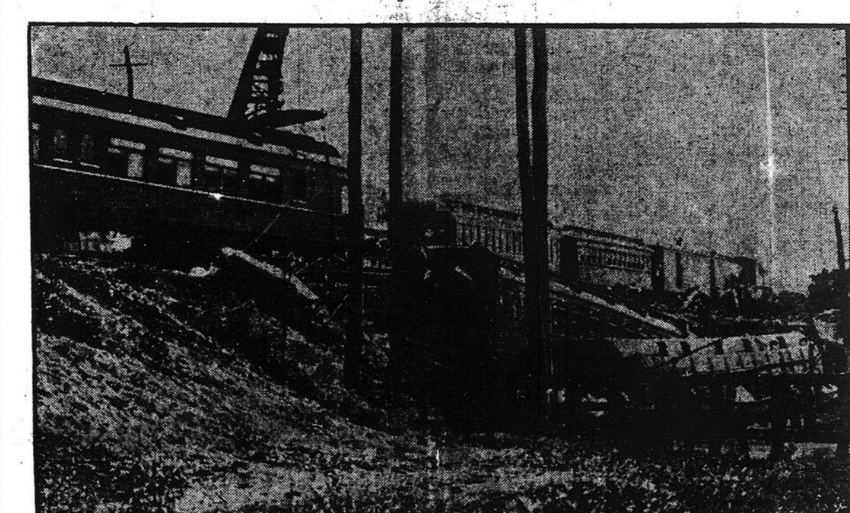
Scene at Bridgeport, Conn., disaster, when the Federal Express, running from Washington to Boston, crashed into an open switch on a viaduct at sixty miles an hour. Of the eight coaches in the train five were crumpled up and debris was scattered over all the neighboring streets. The locomotive was hurled 200 feet. Fourteen persons were killed and forty-four injured.
