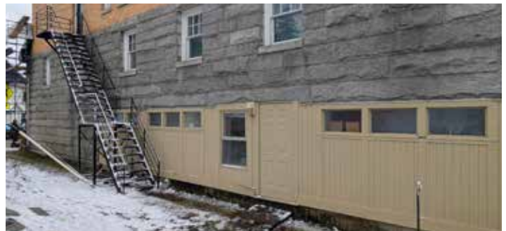
Utility door destined to be new Canadian entrance
