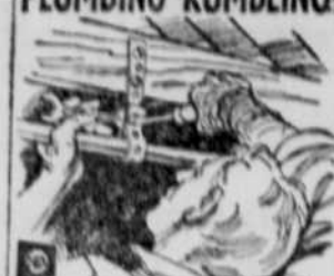
Hanger straps should not hold the line tight against the beam.
