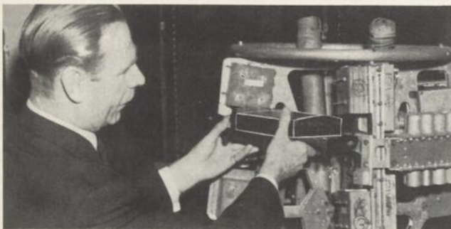
J. S. Brooks, Project Manager, demonstrates how the electronic devices fit easily and compactly into the cruciform internal structure.
