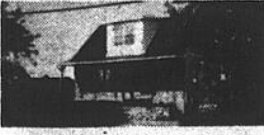
52- SAINT-ALEXANDRE: bungalow, construction 1976, paysager, terrain 22,220 pi. ca. M. Raymond.
