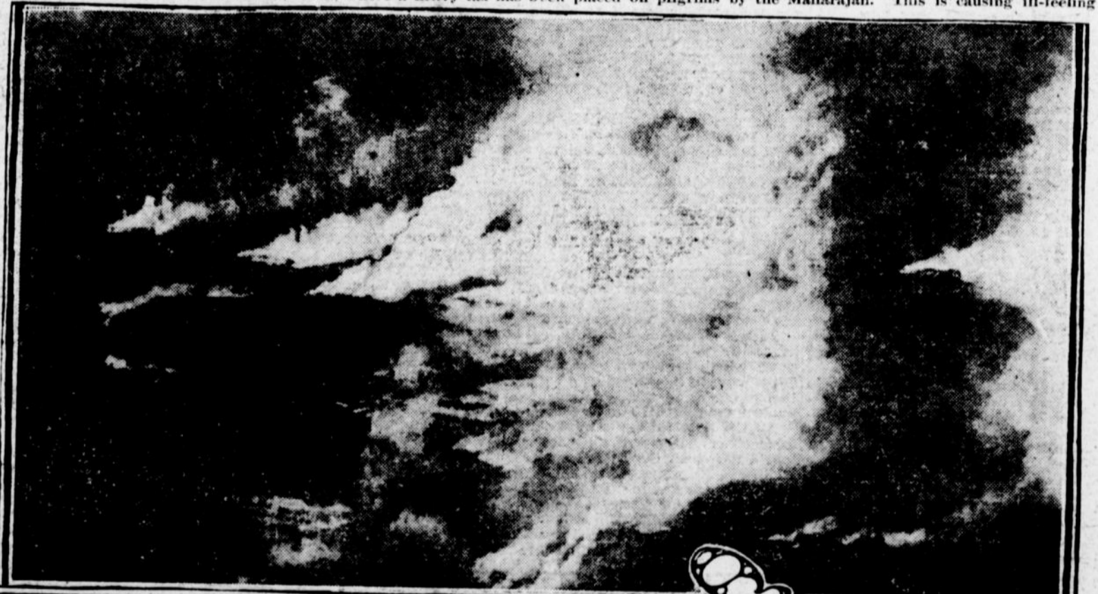
Smoke rising over the ruins of U.S. Naval Arsenal depot, which was struck by lightning recently.
