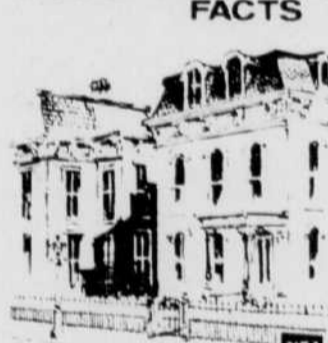
The mansard roof, steeply sloped on all four sides and used as an extra story, was not invented by Francois Mansart or Mansard, after whom it was named. The World Almanac notes that Mansart revived this roof style and gave it vogue during the 17th century. It had been used in the 16th century, especially by Pierre Lescot in the Louvre Palace.
