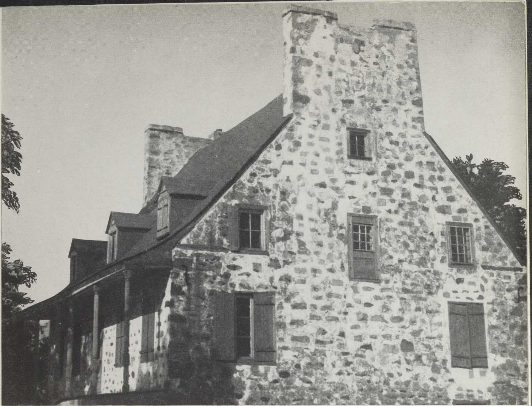
The chimneys and dormer windows are a special feature of the Beauchemin house at Varennes, dated 1770.
