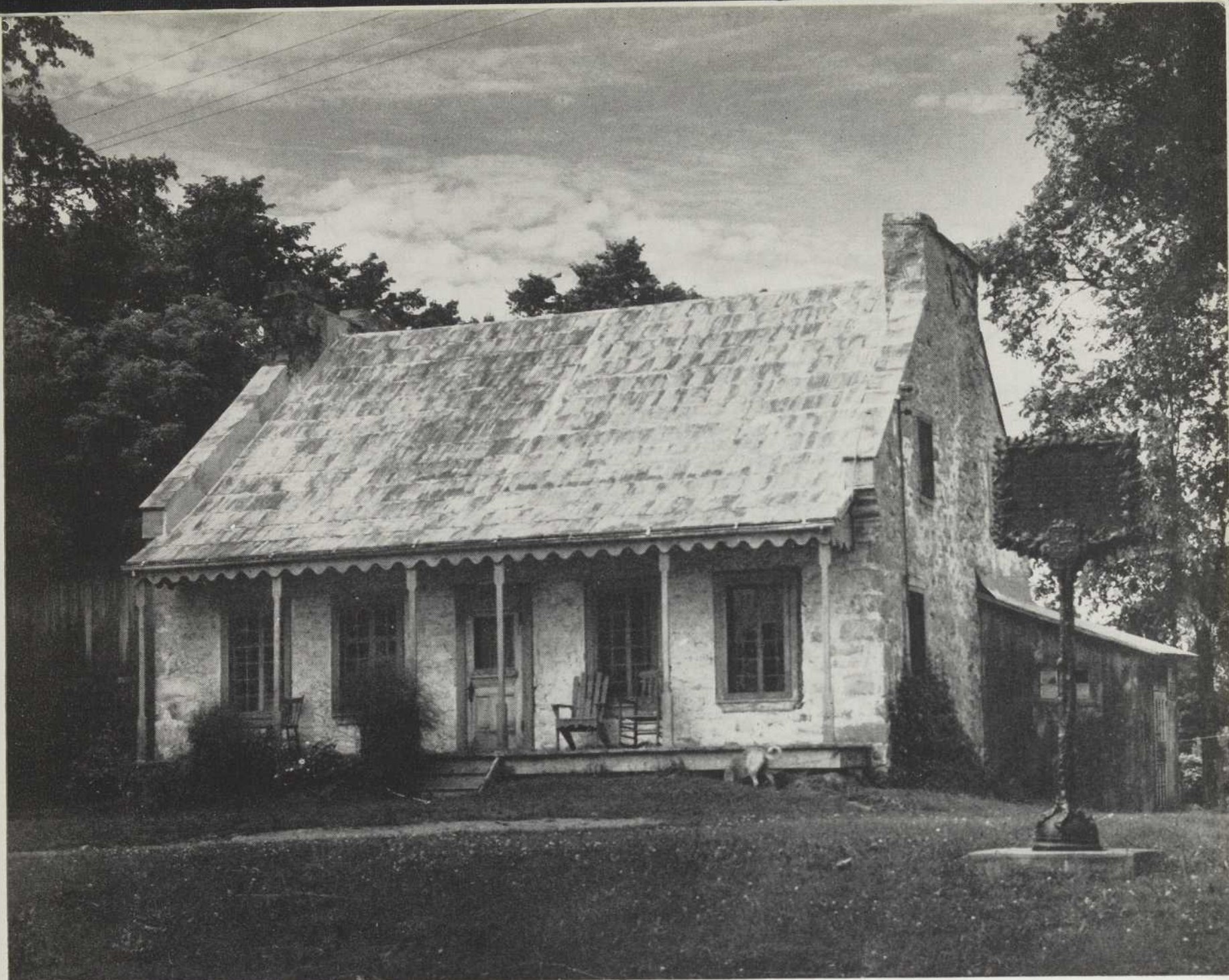
This is the house at Carillon, Argenteuil County, where Sir Adolphe Routhier wrote the poem O Canada. The house shows much good carpentry in its door and window frames.
