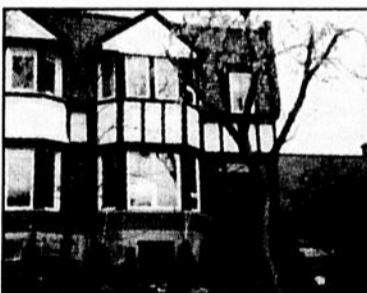
Traditional cottage, high ceilings, great kitchen, 2 car garage. $449,000.
