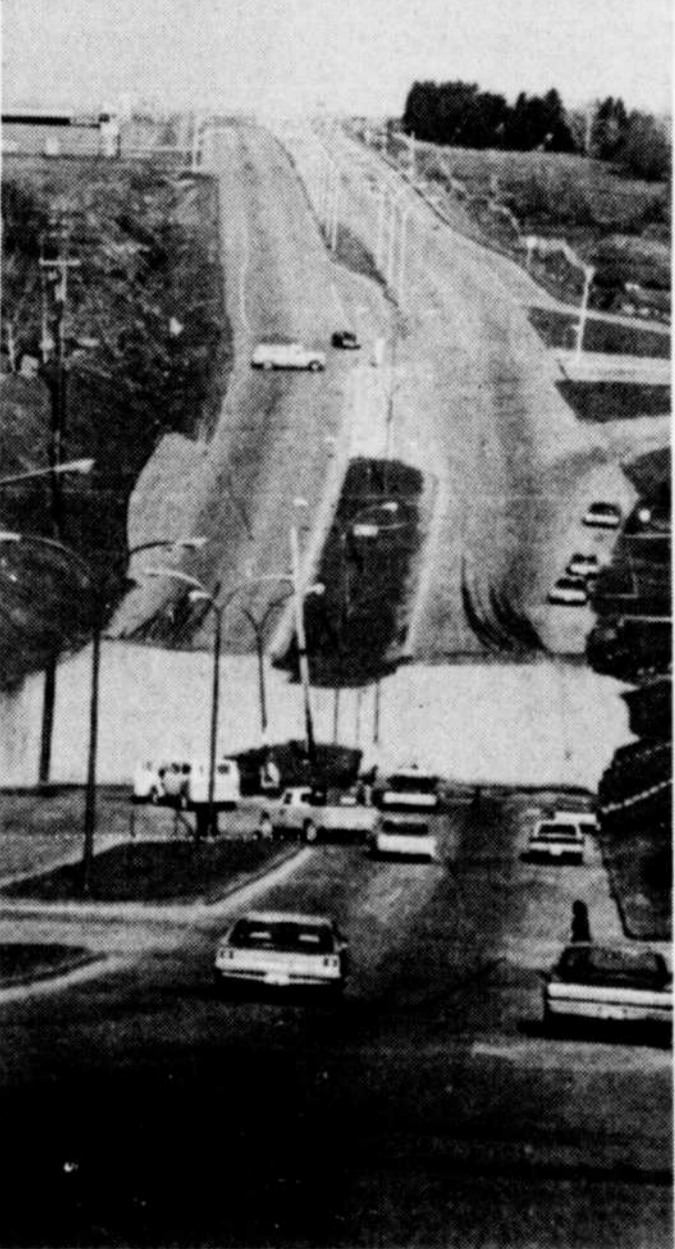
PORTLAND ST. FLOOD — Everyone thought that after the snows melted and the ice went out that flooding in the Sherbrooke area was over for another year. No one counted on a man-made flood yesterday at the corner of Portland Blvd. and Wilson Streets which blocked traffic both ways as a result of a break in a water pipe near the pumping station. The break has been mended and the water pumped away, bringing traffic back to normal on the busy street that runs parallel to King St. (Record photo by Gordon Alexander)
