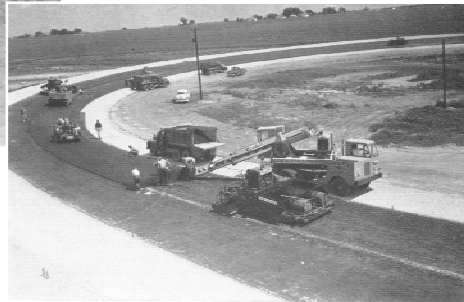
Figure 29. Bituminous concrete construction.
