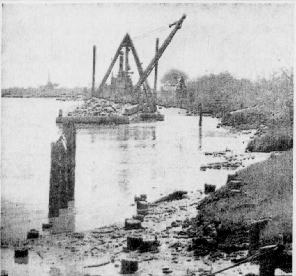
MUDDY SHORELINE — Low-lying Westham Island lies in the middle of the Fraser River, threatened by spring floods from the largest snowpack ever recorded on B.C. Interior mountain ranges. A dredge collects shoring and diking material, which will be used during the spring runoff, expected to reach full impetus in the next two weeks.
